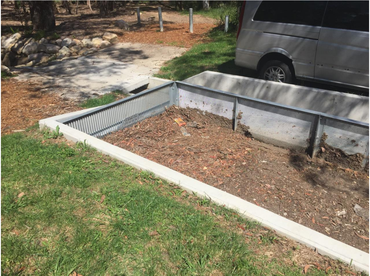
Plate 3 Showing a side view of the Barramy Trap.
